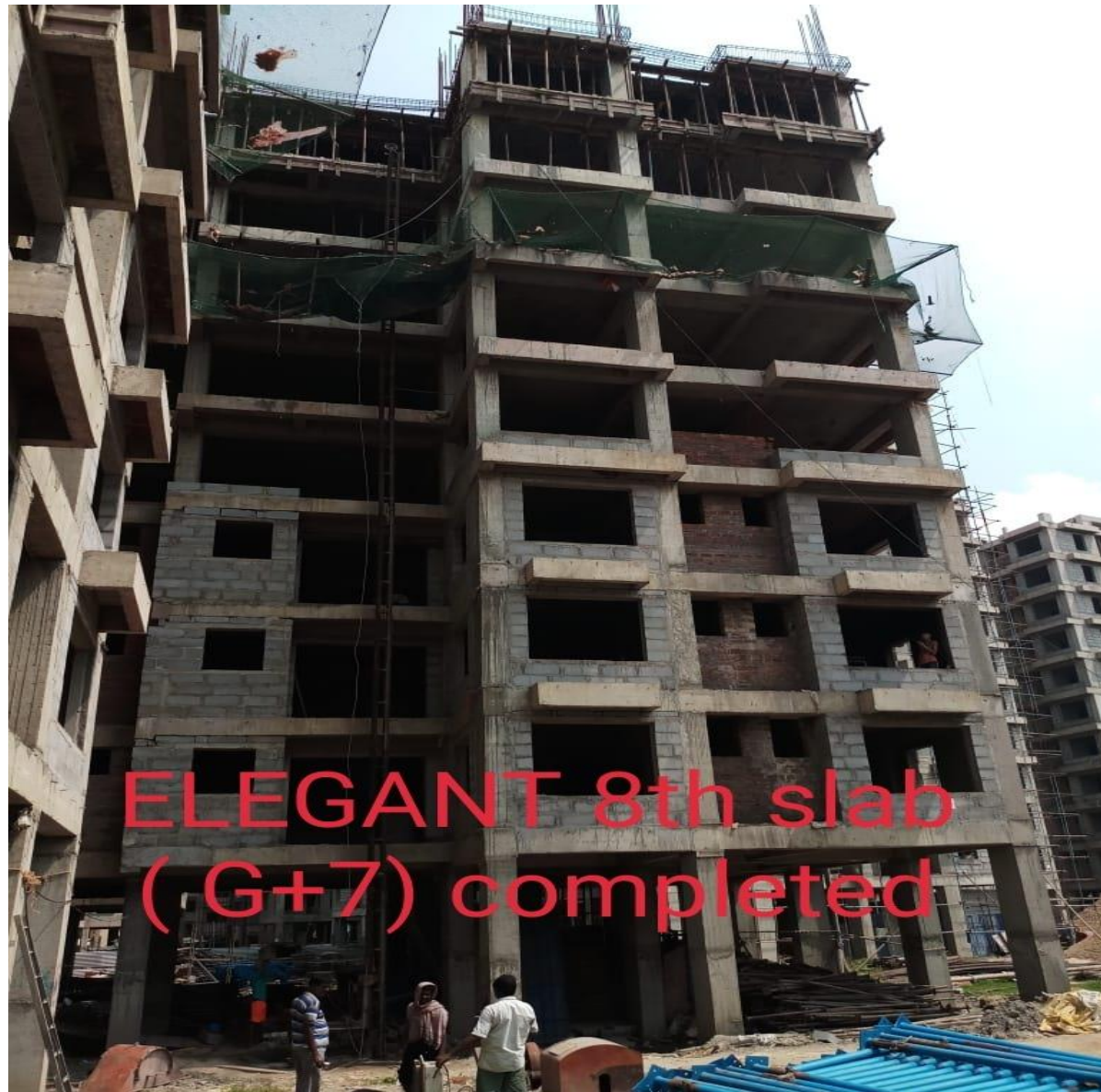
ELEGANT 8th slab (G+7) Completed
