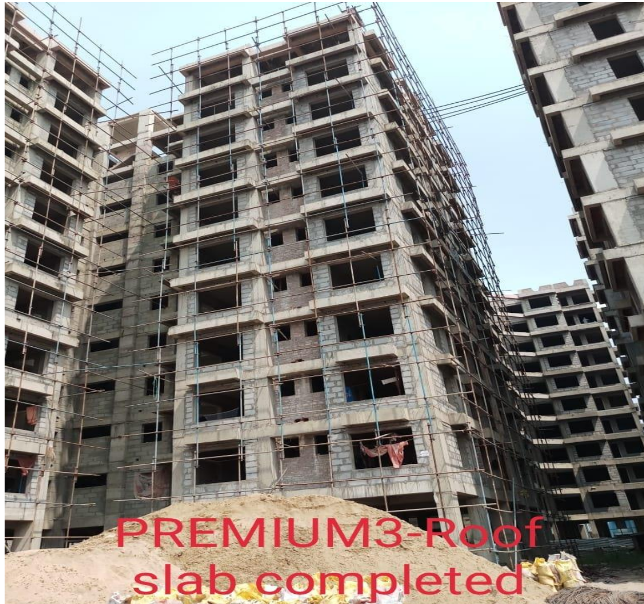
PREMIUM -3, Roof Slab Completed
