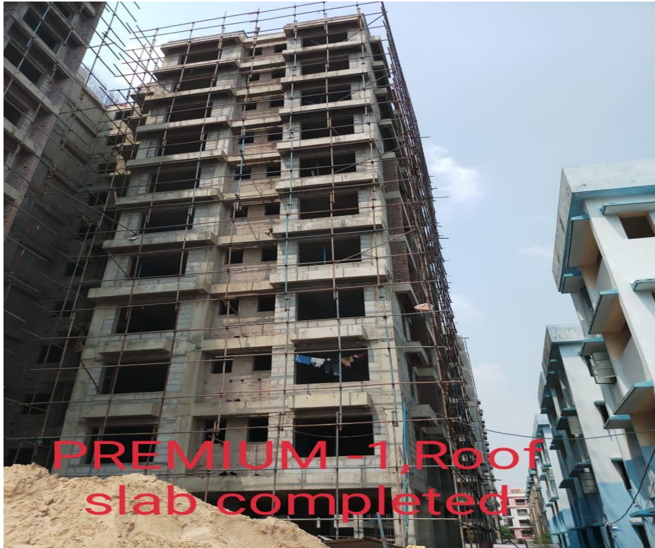
PREMIUM -1, Roof Slab Completed
