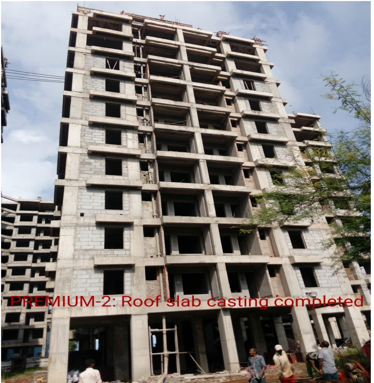
PREMIUM-2: Roof slab casting completed
