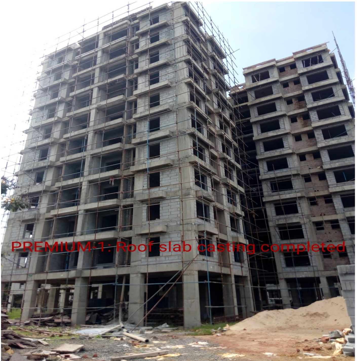
PREMIUM - 1: Roof slab casting completed
